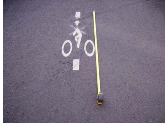
Figure 2. Permanent signal loop detection mark. Place wheels on this mark to get a green!
