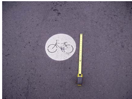
Figure 4. Bicycle Boulevard Marking, not detection marking.
